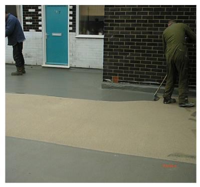
The high-performance products in the Metflex range are capable of being applied by roller, squeegee, notched trowel, brush or sprayer. They are two, three or four component products that from simple coatings to high performance screeds and renders, to a unique range of highly chemical, abrasion and puncture proof elastomeric, high build, instant set spray applied elastomeric membranes.
